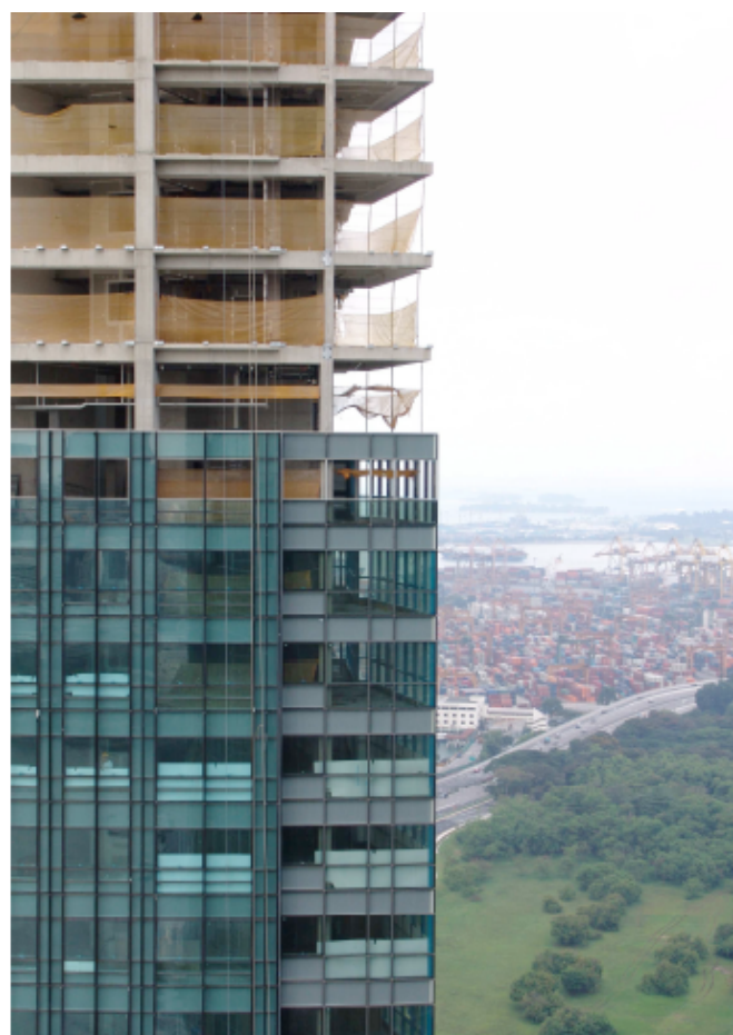
A curtain wall during its installation – a glass skin to the building!
