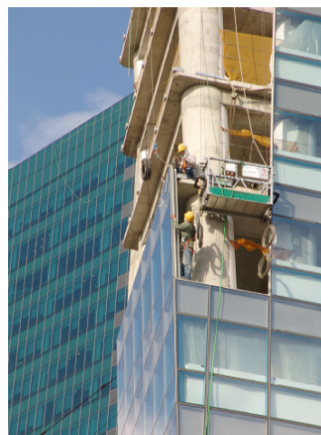
Unitized Curtain wall installation: from left: hoisting panels, using monorail and gondola installation
